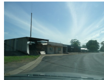
From left to right: Low lying Rocks Ferry Reserve, Fish cleaning facilities, Existing toilet block at top of bank, Existing footpath/cycleway, Disused timber yard above the reserve.
