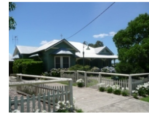
Cottage style with steel roofing
